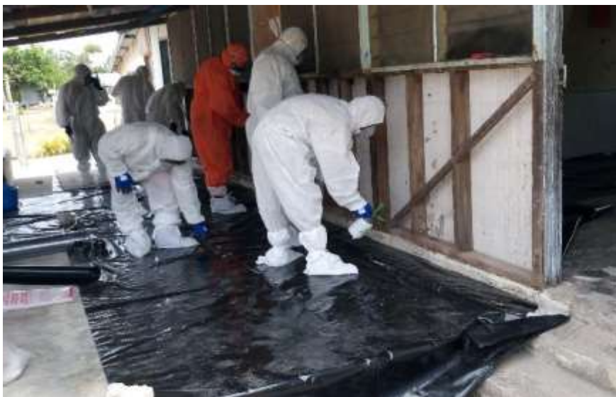
Eton School – Removal of asbestos boards
