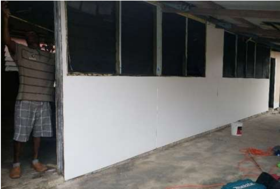
Eton School – The finished job
