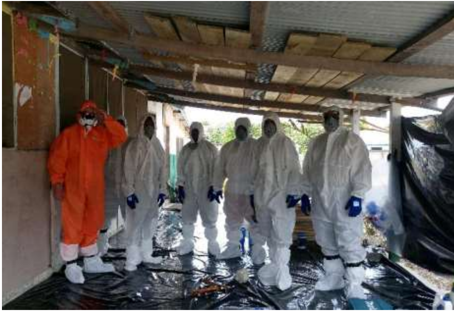
Eton School -Trainees ready to start work
