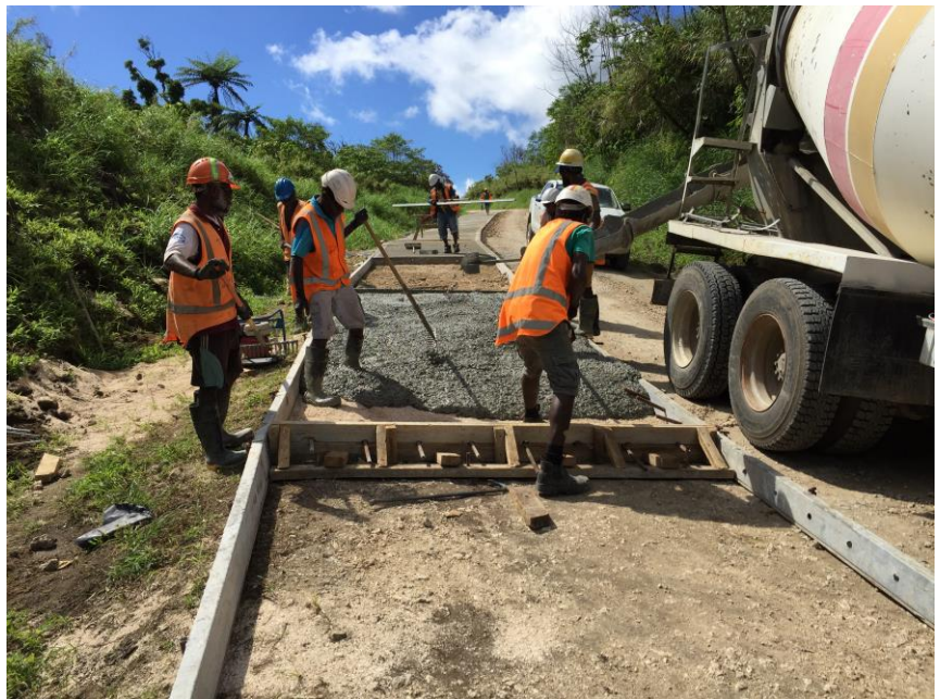
Concrete works underway
